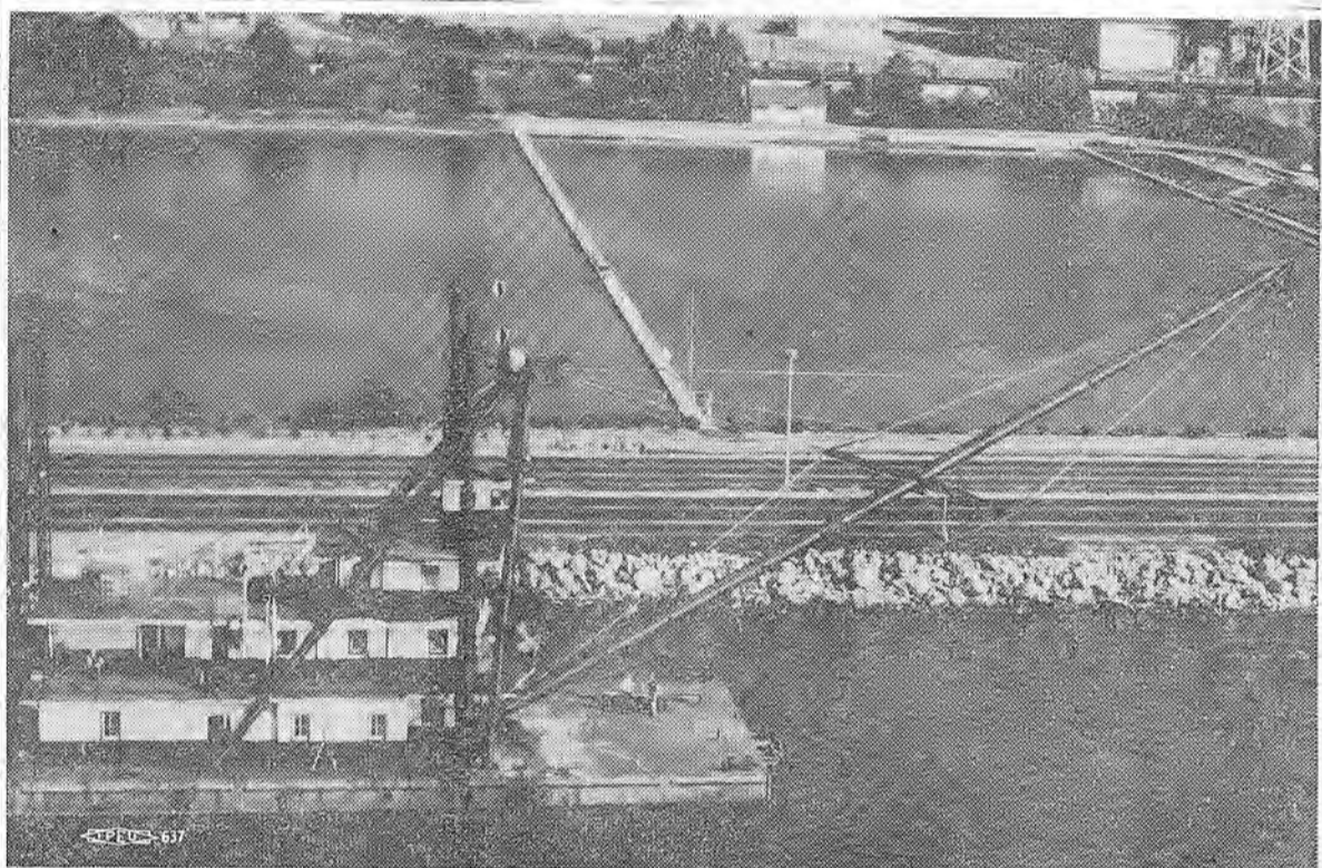
EASTSHORE DREDGING OPERATION —Shown in this aerial view is Simpson Brothers' dredge, "The California," which is again in operation on the dredging phase of the multi-million dollar improve-
