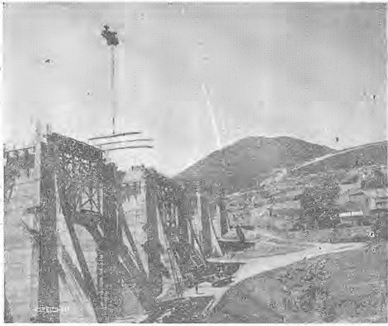
SKY-HOOK DOWN DIEGO WAY—Sutherland dam, a big water project in the hills 42 miles east of San Diego, has lain dormant for 25 years, but now is being resumed, with the need for water. The big concrete buttresses have stood like memorials thru the years. To facilitate carrying of materials to the job, this skyriding buggy on two, 2-inch cables was set up, will carry 20 tons, go 30 miles an hour. Pushing the sky buggy in this picture is Engineer Paul Addison.
