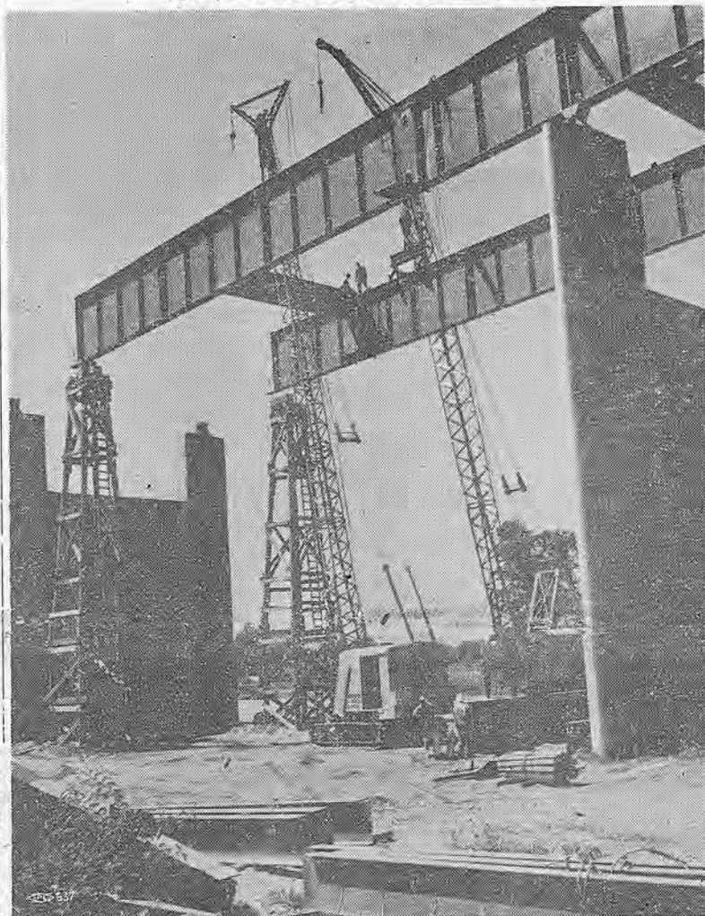
were put in by Parker, and Rice Bros. are furnishing the ready-mix concrete for the deck. It is expected to be completed and open for traffic some time in September.—Marysville report, Bill Waack.
