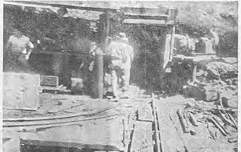
TUNNEL ENTRANCE —This was the scene outside the tunnel following the fatal explosion. (Butte County Sheriff's Dept. photo.)
