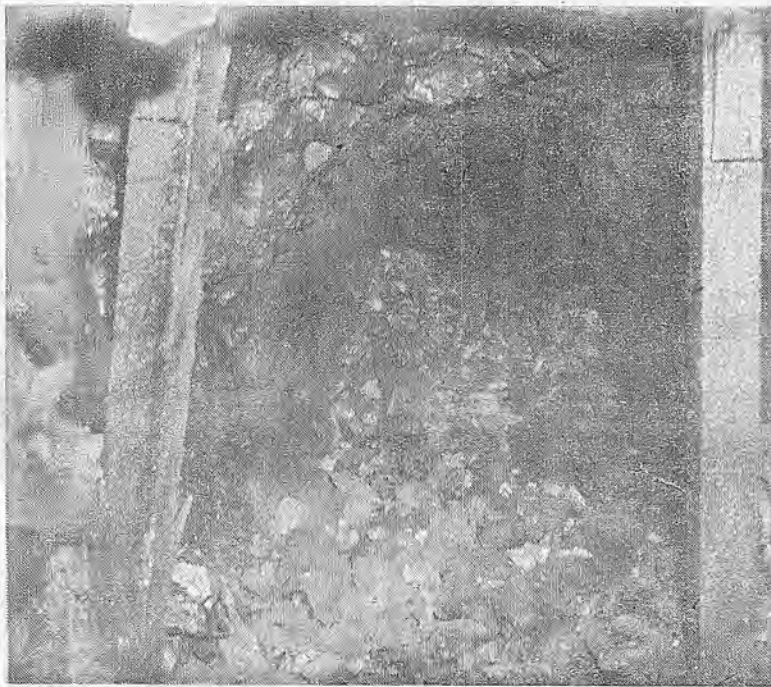
WHERE BLAST OCCURRED —This pile of rubble, deep inside the 1000-foot exploratory tunnel was left by the explosion that took the lives of three men and critically injured Brothers Ship and Canifax. (Picture, courtesy Butte County Sheriff's Dept.)
