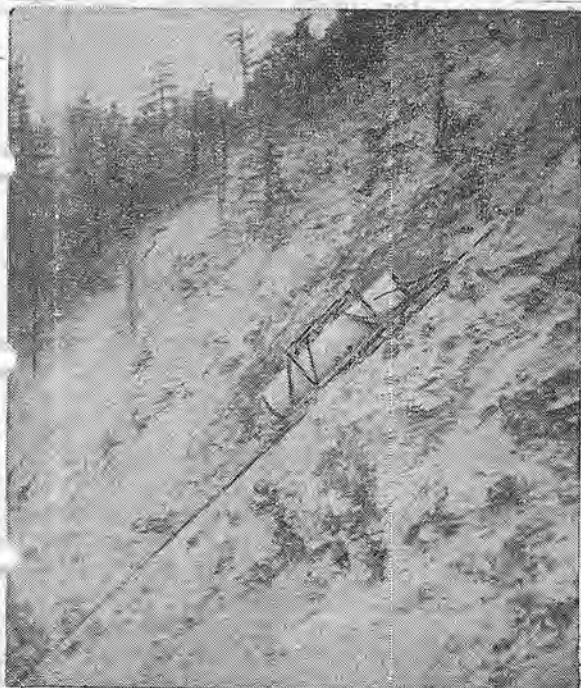
GRUNT PROJECT —The Sierra Nevadas get fairly rugged in many places, but this doesn't stop little man animals from getting the best of steep slopes, hard rock, and rushing rivers. This view shows a heavy lift uphill on the Walsh-Wixson and Crowe Penstock job at Caribou No. 2 powerhouse on N. Fork of the Feather River. (Pic by Bro. F. E. Heisel, Local 3E.)
