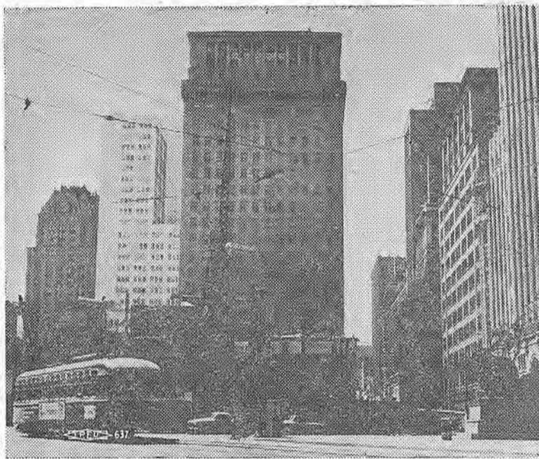
CHANGING S.F. SKYLINE—Operating Engineers are having a big hand in re-shaping San Francisco's famous skyline these days, as several large buildings are underway in the downtown area. This view shows work on the big Zellerbach building at First and Market. Several pieces of equipment are at work tearing down old buildings (lower right), and laying foundation for the new structure. The famed Mechanics Statue, which labor saved from being put out in the bushes at Golden Gate Park, stands prominently at the intersection (lower right).
