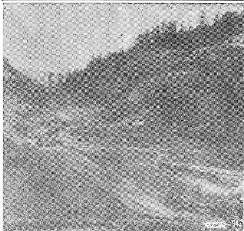
BEARDSLEY DAM SITE.—This view shows the prepared site of the only earth fill dam of the big Tri-Dam project east of Stockton. Dragline in upper right side is working on the spillway and relocation of the Pickering Lumber Co. railroad which will go across the dam when it is completed.
