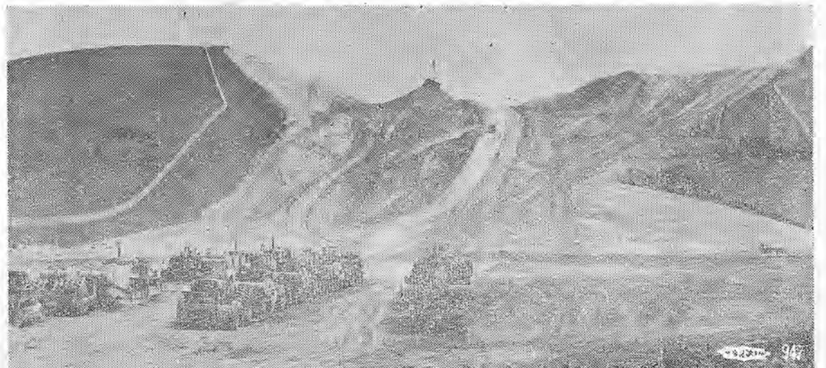
CULEBRA AND CARQUINEZ. —Largest single slice into Mother Earth since the Panama Canal is this 8½ million cubic yard cut at the junction of Franklin Canyon road and Highway 101. It took
