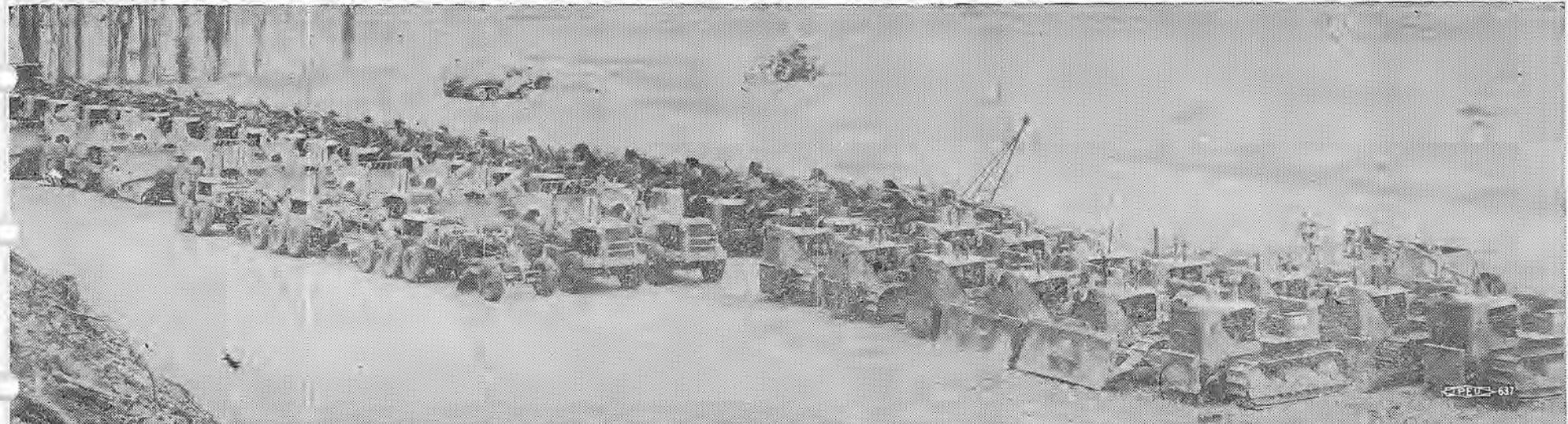
Here is one of the longest line-ups of heavy equipment seen around the Bay in some time. It makes up the total equipment used by Hindry Construction Co. on its four
