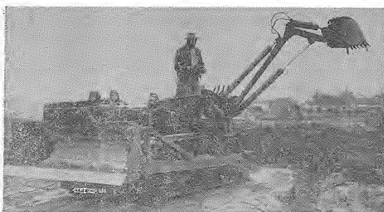
FIRST IN THE WEST in this new Backhoe-dozer combination mounted on International TD-9. It is a honey of a smooth-running rig, has hydraulic action controlling the backhoe. It digs and fills trenches with ease. Proud owner is Operating Engineer I. W. Brooks of Los Angeles.
