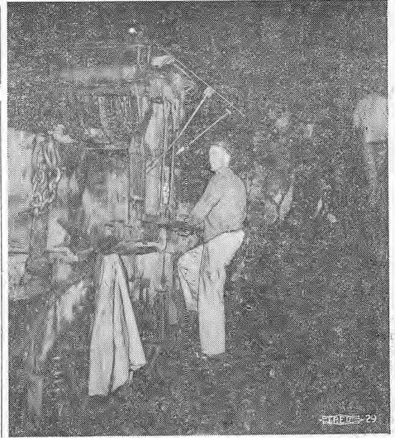
RIDES IT LIKE A BICYCLE —Brother Lester Harles rides this Conway mucker wild West style. It's shown in the lower heading of the Walsh Construction Co. tunnel job at Big Bend.
