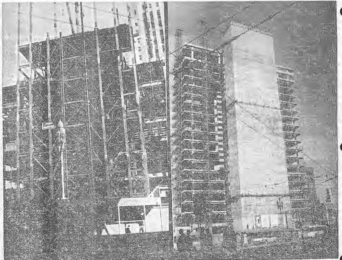
CONSTRUCTION PROGRESS of the Crown-Zellerbach building is shown in two of the photos from the album of Mrs. Johnnie Del Pope, whose hobby is recording the growth of the new, impressive S. F. structures. Picture at left was taken in April 1958, one at right was snapped in December 1958.
