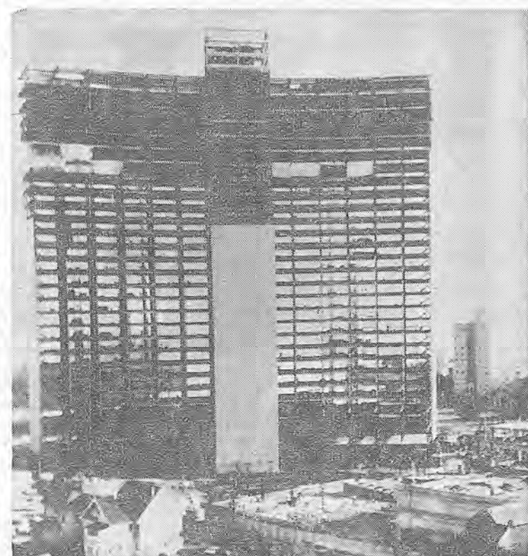
A view of Kaiser Center in Oakland looking east, shows elevator shaft in center of building, shops and garage in foreground. About 80 per cent of building materials are either produced by affiliated Kaiser companies or products made from their raw materials.
