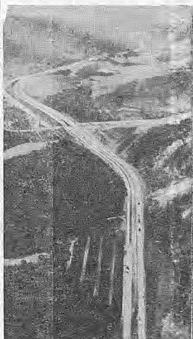
MOUNTAIN FREEWAYS —Moving fast these fine Spring days is work on new mountain highways. Top view shows Sherwin Grade section of U.S. 395 on east side of Sierra Nevada, old winding route in canyon at right. Middle picture shows U.S. 40 plunging its way thru timber near Colfax, pushing fast towards a divided highway over the Sierras. Bottom picture shows the new section of U.S. 50 thru Dublin Canyon, making it four lanes from Oakland to Tracy.
