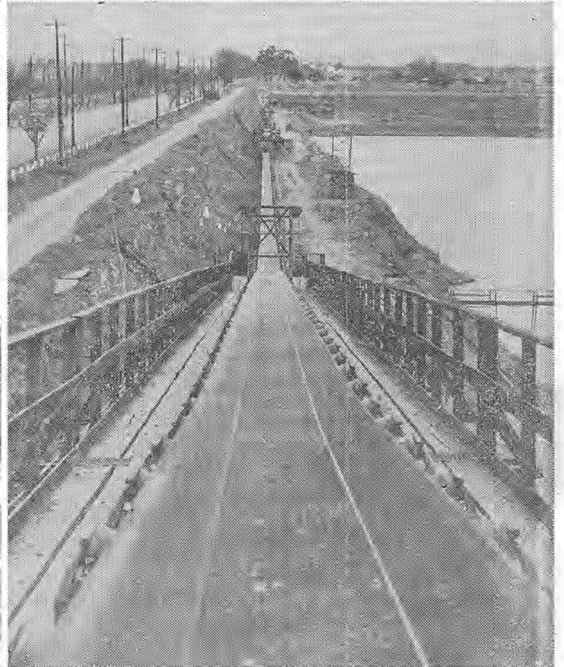
Shown here is a portion of the 7,000-foot conveyor belt at Kaiser Radium Plant which feeds from the classifier to the main hopper of the washing plant. 8,000 tons per day can be put through the classifier. This is the first washing of the pit run at the classifier. The operator on the classifier plant is Charles Drohare, and his oiler is Stanley Rathbone. Charles M. Watt is the mechanic. There are 15 other mechanics in all at the plant. (Picture from Oakland office.)
