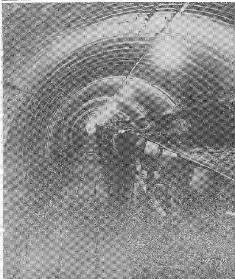
Part of the unique 7,000-foot conveyor belt at Kaiser Radum plant, near Livermore, runs under the main highway and railroad tracks from the classifier into the main plant where material is separated. This one plant ships 25 rail cars and about 4,000 yards by truck, each day. 84 engineers are employed here (Pictures by Bro. Jim Jennings of the Oakland office of Local 3.)
