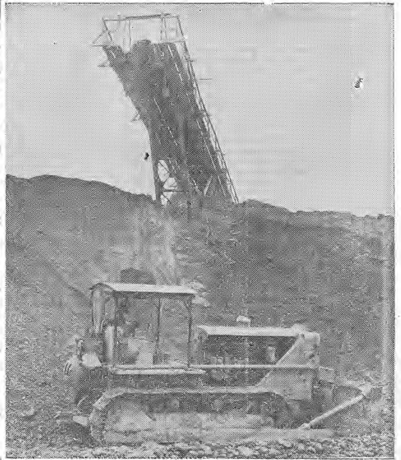
The D-8 cat operator at Kaiser Radium Plant is Arnold J. Cook. This view shows the end of the 7,000-foot conveyor from the classifier. From here it distributes into the main washing plant and is separated into aggregates.
