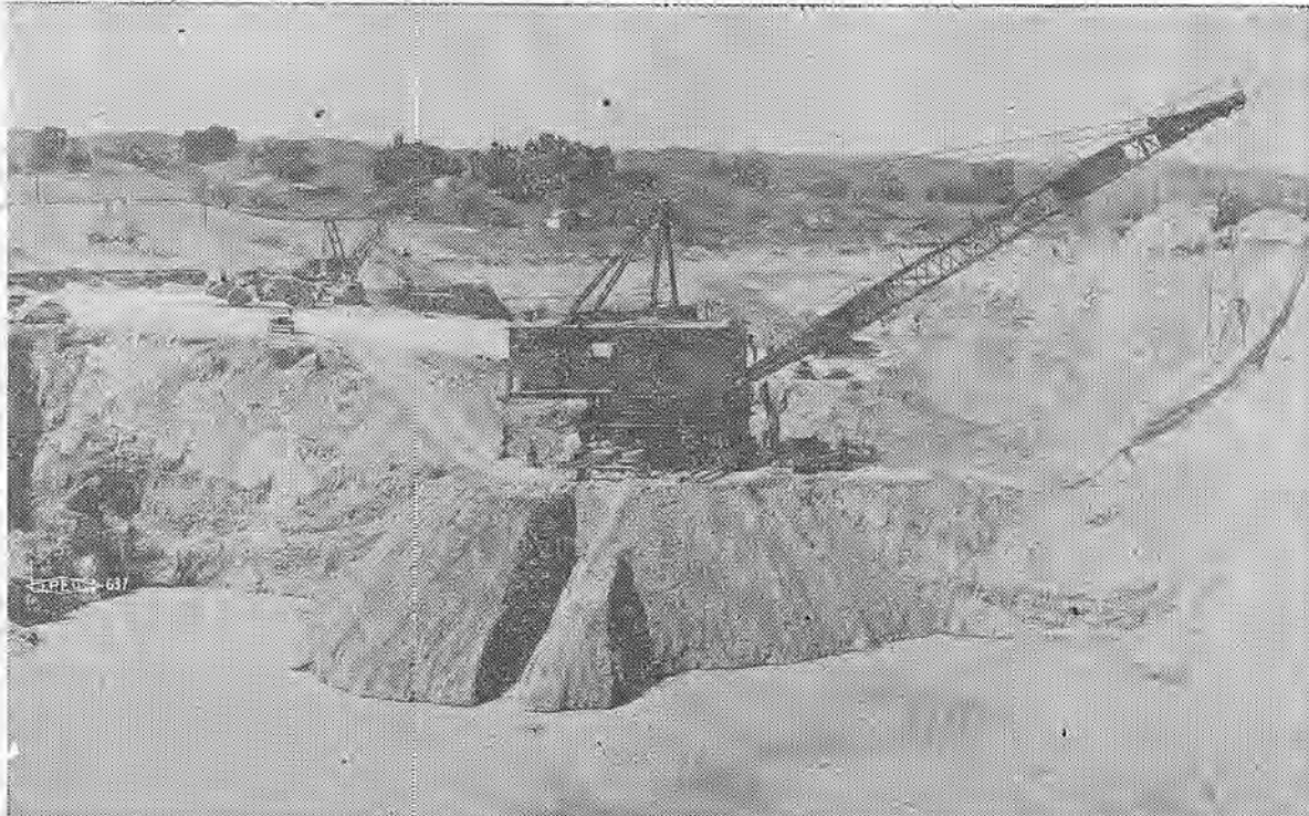
This view shows two Bucyrus rigs feeding the fast-moving Euclids at the Pacific Coast Aggregates Company gravel pit. These giant rigs are manned by Operating Engineers, with several hundred employed in the Southern Alameda county plants.
