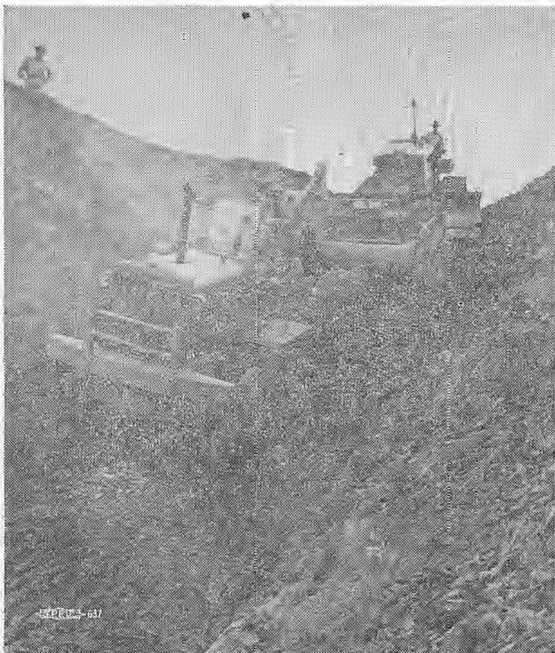
Big rigs lay groundwork for the approach to the new Northbay bridge from Richmond to San Rafael. Walsh Const. Co. DW20 is shown here operated by Operating Engineer Cliff Bakewell, and behind him on the Push Cat is Harold Corbett.
