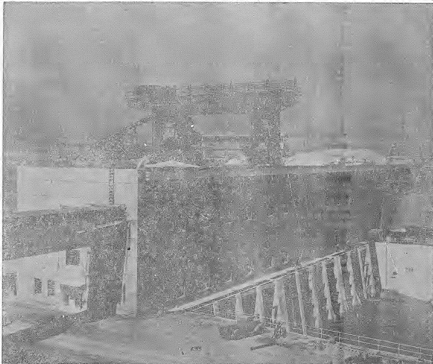
From this giant pumping plant near Tracy, California, water flows uphill. Six 22,500 horsepower pumps actually lift two million gallons of Sacramento River water per minute a height of 200 feet into the Delta-Mendota Canal and thence into the parched San Joaquin Valley.
