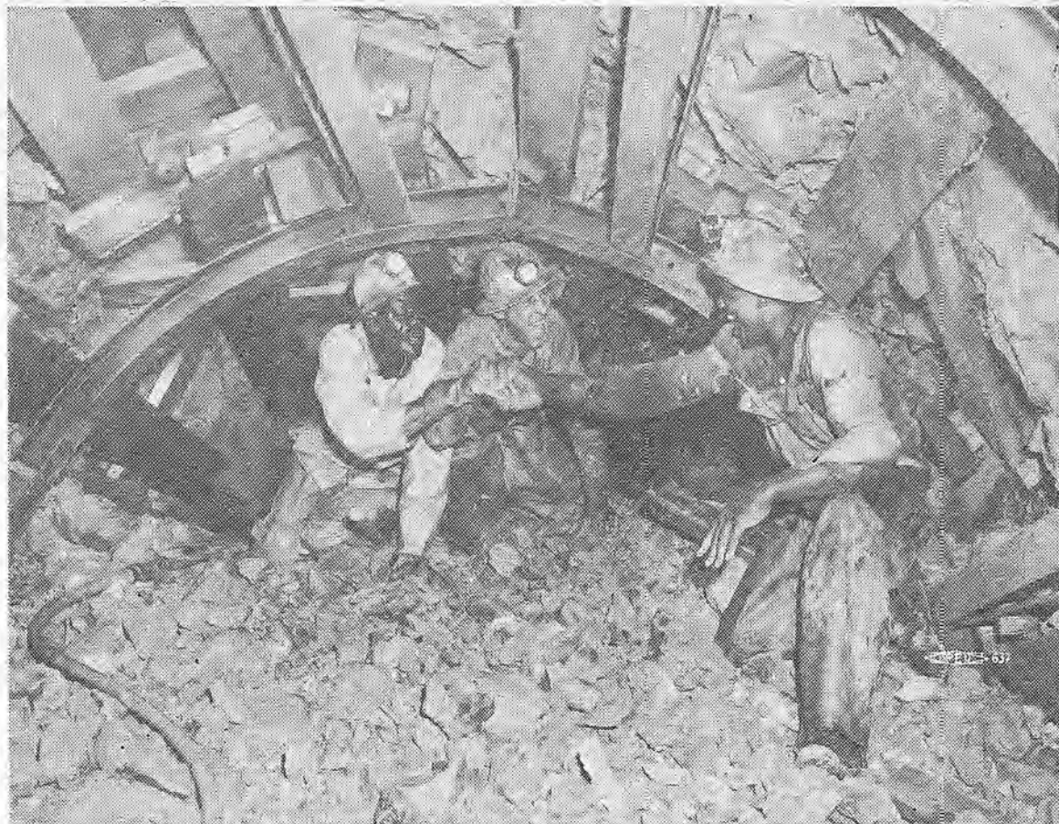
HOLING THRU, ON THE NOSE —These boys reflect the happiness of water company and contractor officials on the accurate meeting of two bores on the San Francisco Water Company's tunnel project after 13 months of boring under the city of Hillsborough by Peter Kiewitt Co. (Story on page 2)
