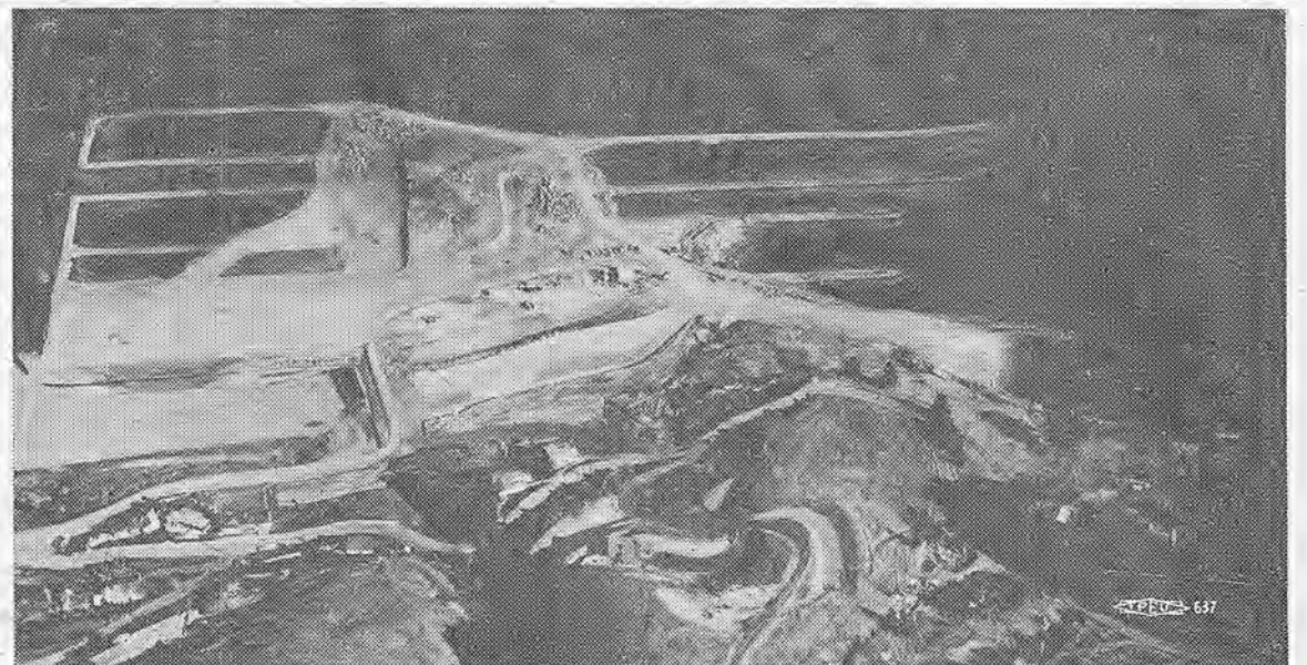
RE-SHAPING SAN FRANCISCO BAY —Rocky piers form hollow rectangles which will be filled in solid to create Paradise Cay home-building development on the Belvedere Peninsula in Marin county, being built by Pullman Bldg. Co. Fills go as deep as 50 feet. For an idea how the finished product will look, see picture on page 3.
