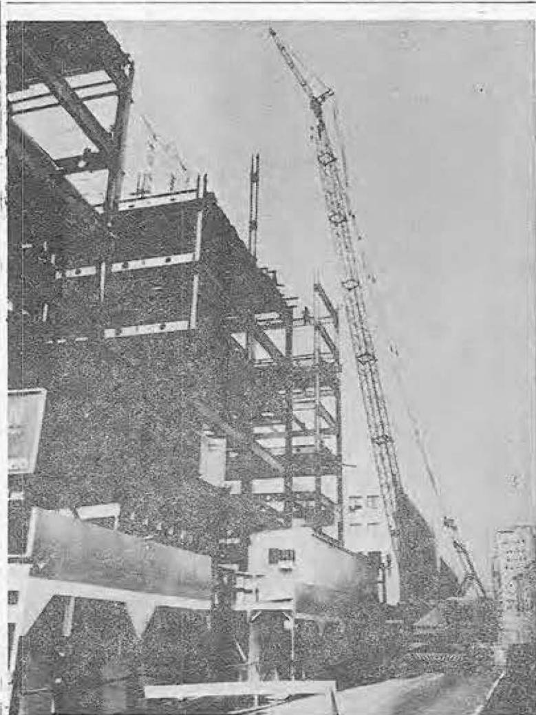
SPECIAL DELIVERY —First building of 13-story height where all steel was set by a truck crane rather than the usual stiff leg derrick, etc., is the So. Calif. Gas Co. building at 8th and Flower in Los Angeles. Here the Heisler and Woods crane is shown working on the 8th floor, using 180 feet of boom and jib. Prime contractor is Lindgren and Swinnerton, Inc. View is looking west on 8th street.
