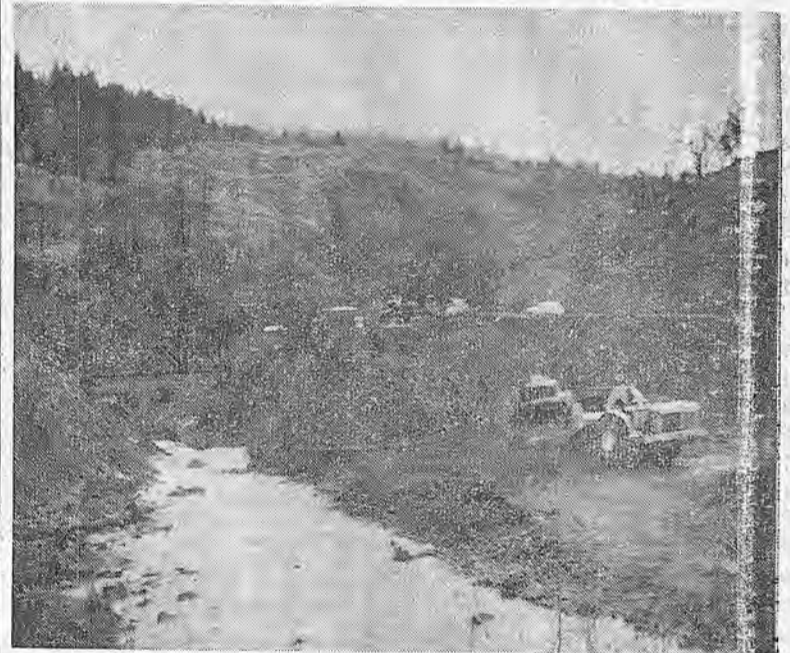
WINTERTIME JOBS—Up until the second week in February at least it has been one of the mildest winters on record, making it possible for many contractors to continue work, whereas normally they are shut down tight. This picture shows work under way on Thomas Const. Co. bridge and road job seven miles east of Longvale which is just north of Willits in Mendocino county. A new bridge and road-straightening are due here.
