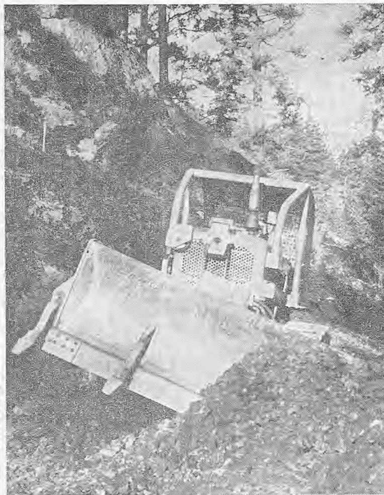
A D7 equipped with No. 7G Gyrodozer pioneers a construction road in rocky soil in the Sierras. Teeth attached to moldboard fracture rock in advance of dozer blade. Tip and tilt of blade are accomplished thru use of hydraulic cylinders mounted to draft arms. The Gyrodozer is proving itself in a variety of applications for rough materials working.
