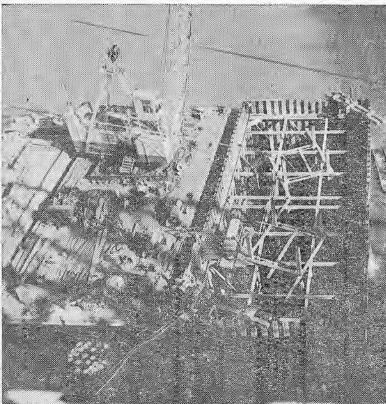
PIER 4 is a different type of construction. It is just off shore near the C&H sugar plant on the Crockett side. This view shows concrete being poured by a Smith-Rice rig. Inside forms are built inside of sheet piling driven for this pier's form.
