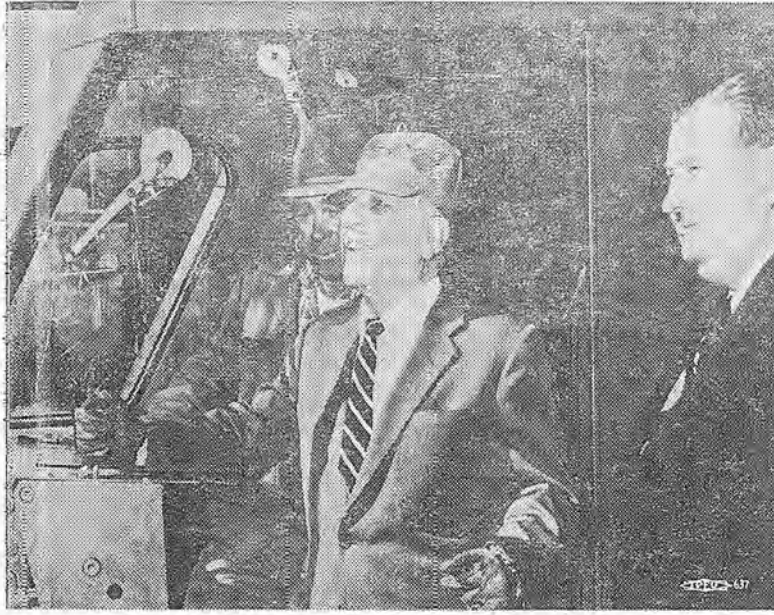
GOVERNOR-ENGINEER. —Gov. Goodwin Knight, honorary member of the Operating Engineers, gets final operating instructions from Bro. Geo. Haskins as he takes control for first pass at one of the old buildings being demolished in Sacramento's clean-up program. Assisting the governor is City Councilman Al Marty. Oiler on this rig is Bro. Joe Mannos. (See story, picture on page 5.)
