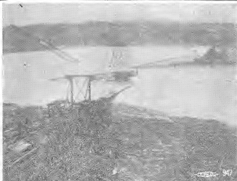
BAY AREA FLOOD SCENE—The Bay Area got its share of the Christmas deluge, as this view of the Kaiser Radium Plant pit near Livermore shows. Note 5-W Draglines, well submerged. It is taking about five weeks of pumping to clear up the accumulated 100 acres of water.
