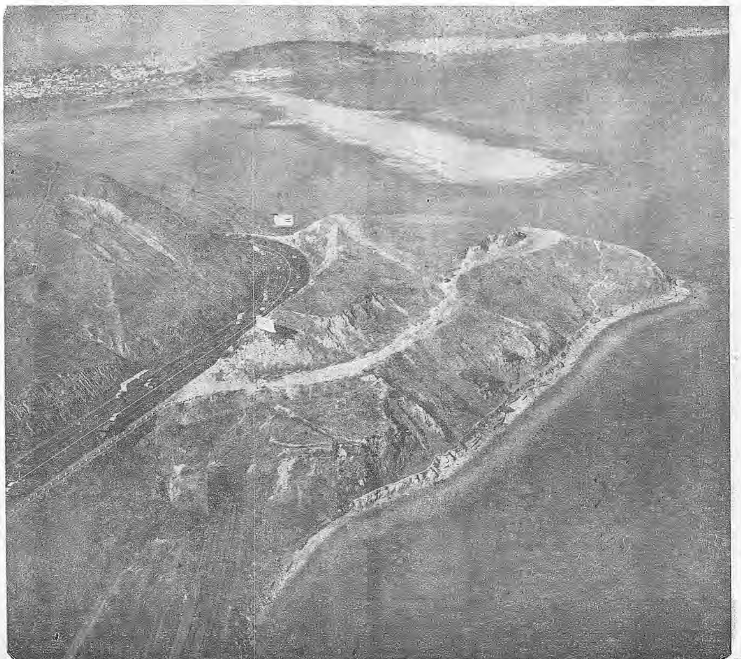
FLOOD TIME ON THE FEATHER —These are before and after views of the Christmas flood damage on the big Poe Tunnel project of Utah-Bates & Rogers for PG&E on the Feather river about 70 miles north of Marysville. Upper picture shows work in progress before high water, and lower shows how most of it disappeared. The 34,000-foot, $15 million tunnel job was badly flooded out on the intake portal, throwing men out of work, but as the damage is cleared away operations are getting back to normal. The tunnel is part of a $45 million PG&E power project at this location, a sizable addition to the north-state's booming hydro-electric and water conservation program. (Photos by Wes Collett.)
