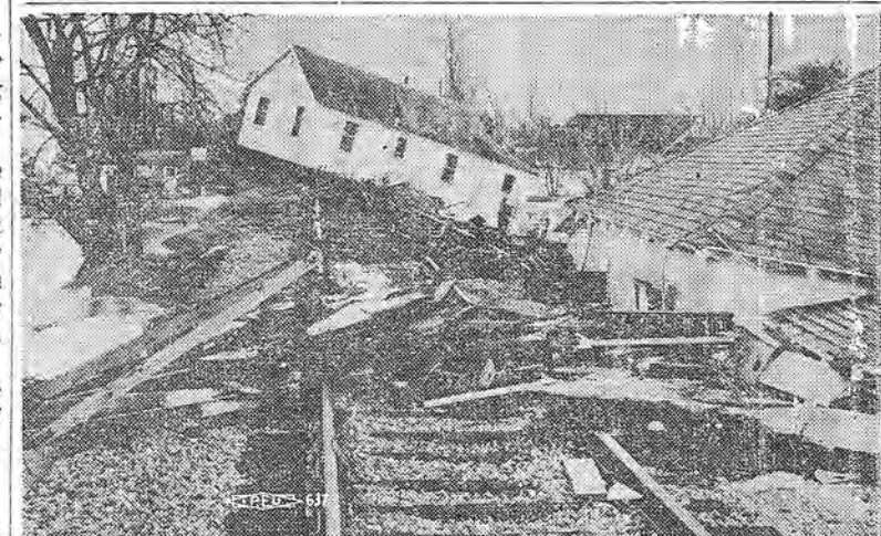
YUBA CITY was hardest hit in the Christmas flood, as this view of two houses cramping a railroad line, demonstrate. Restoration work is now in full swing.
