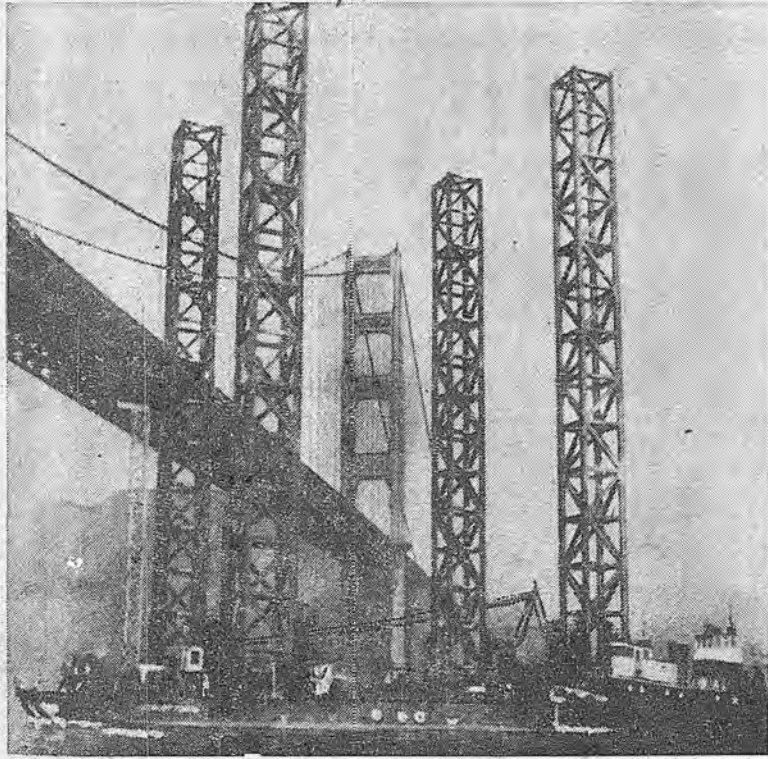
SEA LEGS —The 275-foot legs of the world's largest offshore mobile barge, the "George F. Ferris," were lowered to clear the 232-foot high Golden Gate Bridge on Dec. 15. Then they were jacked up to clear the Gate sandbar, then lowered to 37 feet to give ballast for the 5-day journey to El Segundo, near L.A., to lay six miles of giant sewer pipe in 200 feet of water.
