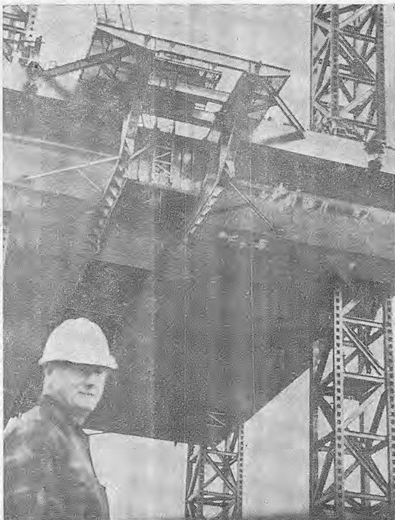
SEA GIANT —This 6,000-ton rig will build Hyperion sewer near L. A., then do offshore oil drilling. 25-story legs are jacked up or down by 3 motors in each at 40 feet per hour. Two tugs nudged it from Richmond out the Gate and down-coast in mid-December. Man at bottom is Rod Chisholm, jobsuper. Picture was taken at Richmond just prior to floating and departure of the unique vessel.
