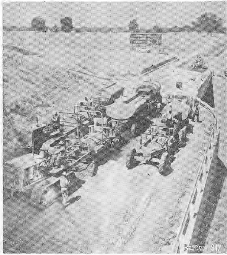
FAST FREEWAY OPERATION—Shown here is the largest cement treated base operation in the world—three Petti-Bone Woods Mixers operated by Miles & Son Co. on the Baldwin freeway job located at Roseville. These mixers average 6500 feet per day and have now completed this operation. Bro. Bud Obenosky was in charge of this entire project. (Picture from Sacramento office.)
