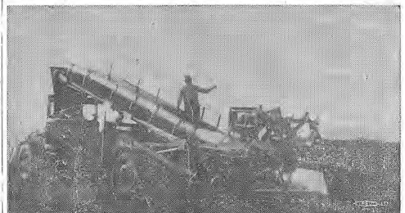
ANY OLD ROADS FOR SALE?—An unusual job of re-processing asphalt roads laid many years ago is being done by this Athey Force Feed Loader and Serria Crusher operating at Orange County Airport.
