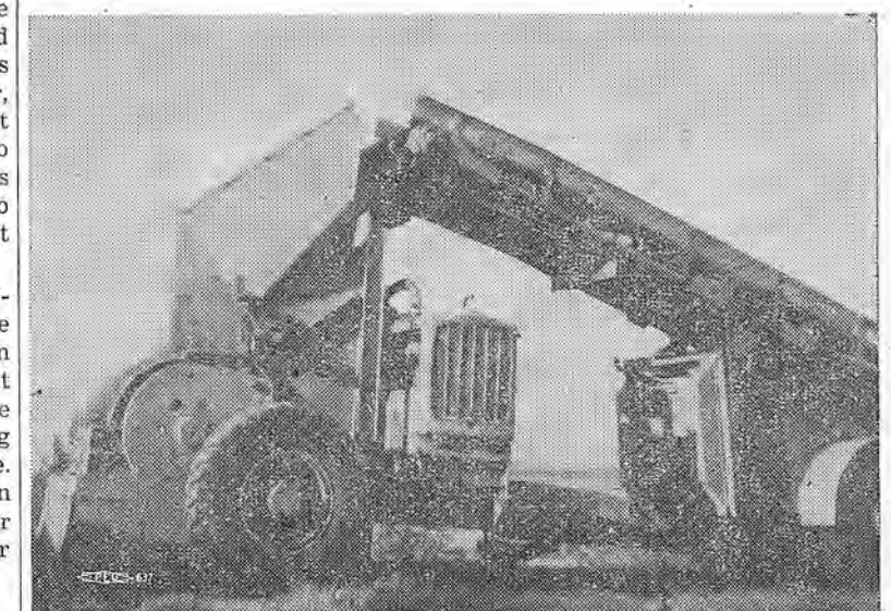
ASPHALT RE-PROCESSING —Here's another view of the unusual Athey Force Feed Loader and Serria Crusher operating at Orange County Airport, re-processing asphalt laid many years ago.
