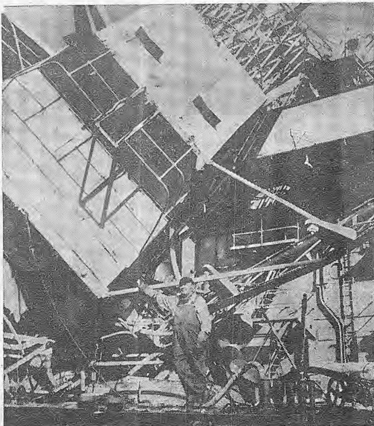
FAREWELL TO BATTLEWAGONS as we go into the age of faster, lighter surface ships. The torch is being applied these days to the USS Maryland at Todd Shipyard in Alameda. Here a workman leans against the giant control tower, which has just toppled.
