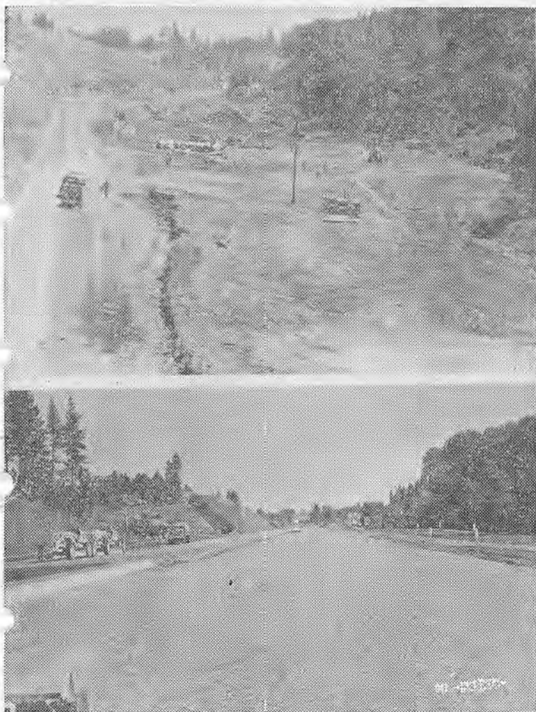
BEFORE AND AFTER. —Here are two views of the same section of Highway 40 in the mountains east of Sacramento. This is a McCammon & Wunderlich job, started Nov. 14, 1956 and nearing completion. Pictures were taken at Bisschops restaurant. Project manager is John New; superintendent, Pat Stewart; foreman, Carl Gentry; crew Ed Bridges. Bob Stanley, Bill Thompson. Another job well down by Local 3 members.
