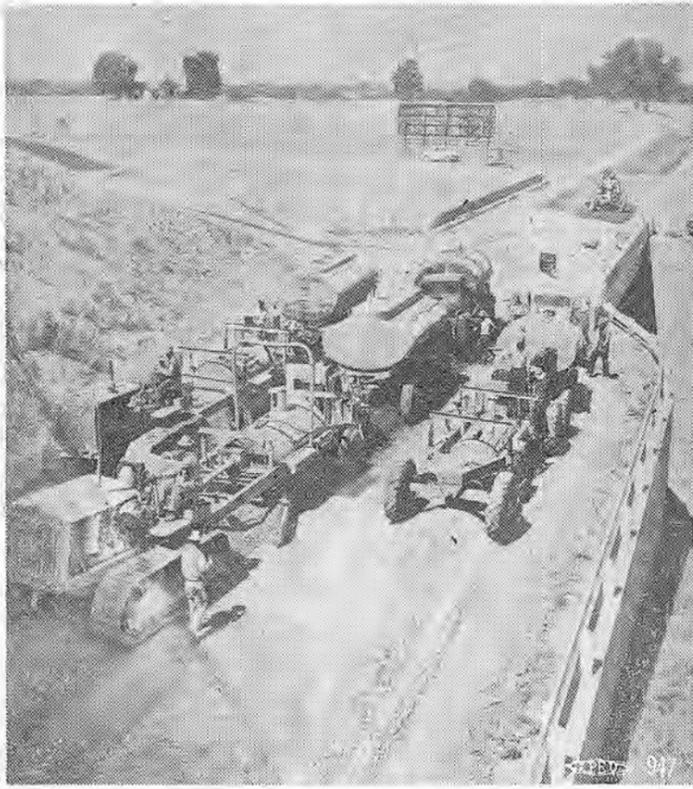
**FAST FREEWAY OPERATION**—Shown here is the largest cement treated base operation in the world—three Petti-Bone Woods Mixers operated by Miles & Son Co. on the Baldwin freeway job located at Roseville. These mixers average 6500 feet per day and have now completed this operation. Bro. Bud Obenosky was in charge of this entire project. (Picture from Sacramento office.)
