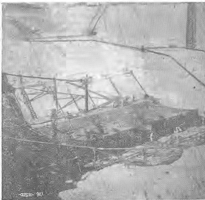
Operating Engineers go to all manner of strange places in their work, and this spot 90 feet below the desert floor is no exception. It is the foundation for the hydro-electric plant on the All-American canal at Pilot Knob. Material is unloaded by gantry crane from flatcars. Generators alone weigh 89 tons.
