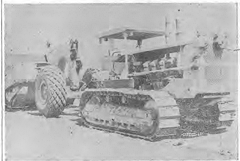
HERE'S 227 HORSES chained up in a V-8 cat that is in operation by a cemetery association in the southern part of the state. The 27-tonner gets up to 250 hp. It has a thousand hours of good operating to date, and Operating Engineers running it say it's the best balanced rig they have ever used.
