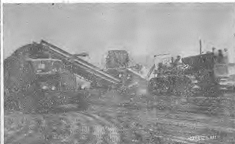
EVERY 43 SECONDS A LOAD—That's what a Sierra Loader, powered by caterpillar motor and pulled by D-8 Cat, leads on semi-dumps, and with truck and trailer it is one each minute. This is on an Atlantic Constructors freeway borrow pit in Southern Cal. On the job are Bros. Alex Braemonte and James Autrey.
