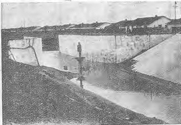
Considerable damage was incurred in the season's one big rainfall recently at the San Lorenzo Creek flood control project of Gordon Ball Co. Pictured are stilling basin and slope paving where water was deepest.
