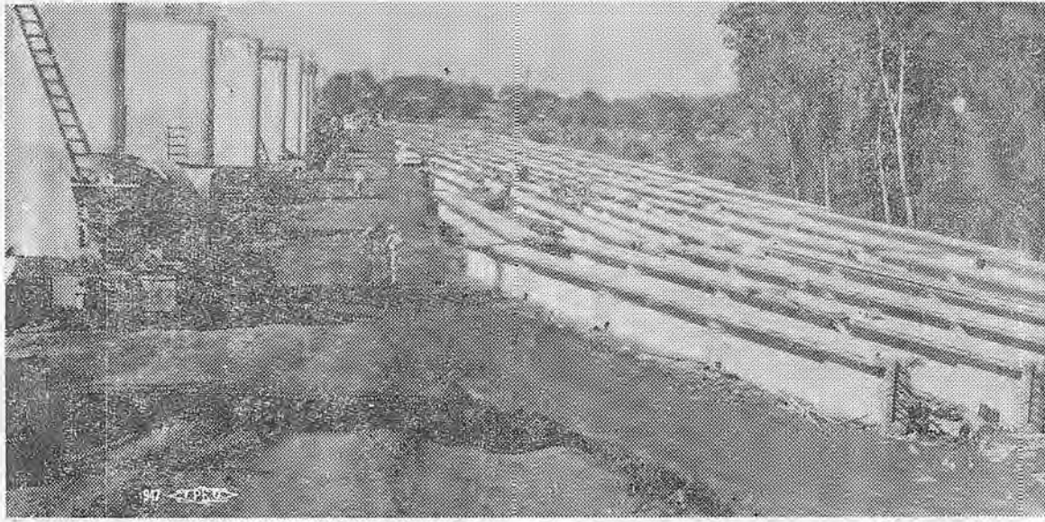
ACRES OF GIRDERS — Pushing fast to beat the rains is this Yuba City-Marysville bridge to replace the one erased by the flood. The many girders at right are pre-stressed concrete. (Photo by Les Collett)
