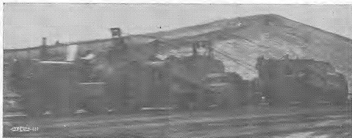
HIGH-BALL 88 TONS —This DW-20, pulling a scraper, moves along at 45 mph on the big Carquinez cut, huge Ferry Bros. and Crow excavation. The load is 48 tons, the equipment, 40 tons.
