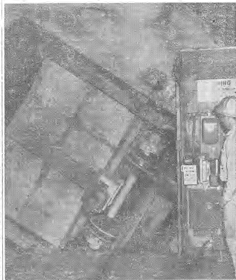
ROLL ME OVER —Bro. Hilmer Felton, member of Operating Engineers Local 3, is shown here running the "rotary dump" at Addit No. 1 of the Utah, Bates & Rogers contract on the huge PG&E Poe tunnel and powerhouse project in Feather River canyon. The "gadget" dumps a carload with ease. (Pic from Marysville office, Local 3)
