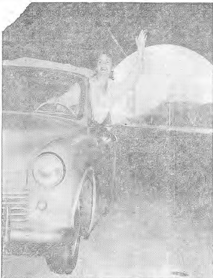
REDWOOD EMPIRE BOUND — Pretty Sandy Teboe drives through the new $1,750,000 Waldo Tunnel, now open to north-bound Redwood Empire traffic. The new tunnel soon will handle two-way traffic while the old tunnel and approaches are being reconditioned. In the background is the Golden Gate Bridge whose tolls will be reduced on Oct. 1, the second slash in 1955.
