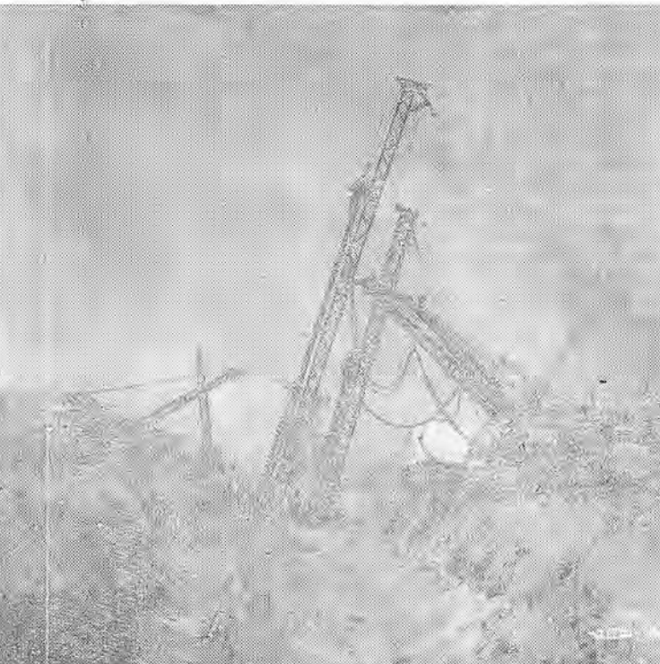
ENGINEER DENTISTS —Doing a lot of drilling, with specially-built rigs, courtesy Kiewit Company, are the brothers on the big Ramona Freeway job at El Monte. Kiewit got the job at $6 million, largest single contract in state history. More than 4600 piling are being driven, and drillers, with pressure pot and hanging leads, are built around a 22-B Bucyrus Erie Crawler Crane, a Northwest Model 25, and a Northwest Model Six.
