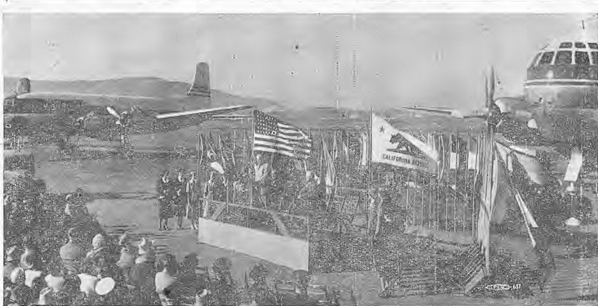
Above is a view of the groundbreaking ceremonies for the new $6,775,000 terminal at the San Francisco Airport Oct. 5. The event
