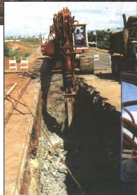
Clifford Cox, on an excavator with a ho ram, concentrates on his work at Royal Contracting's drain line project in Kunia Village on Oahu.
