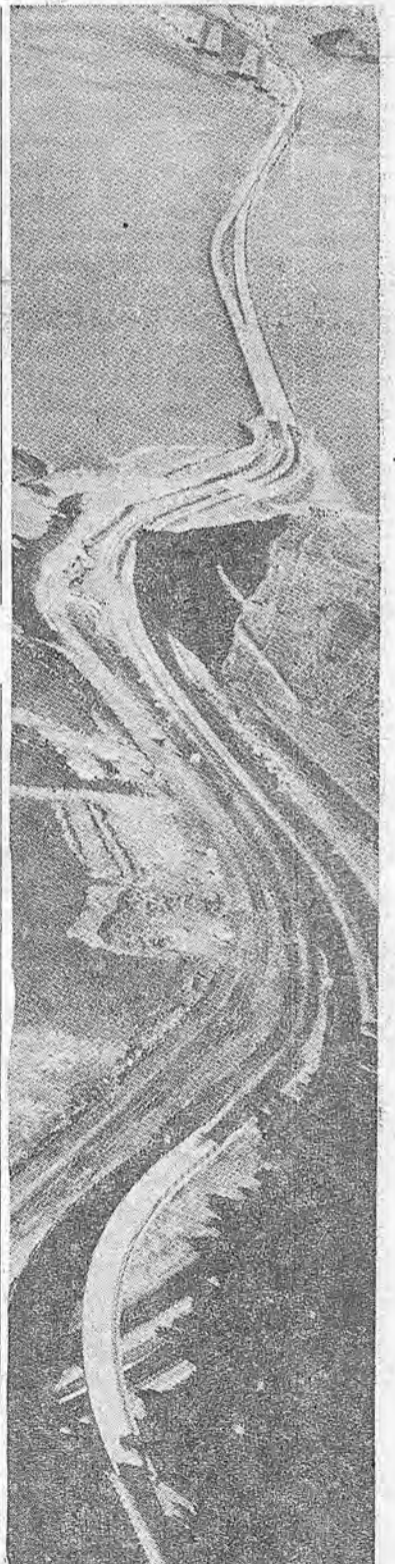
PATTERN OF PROGRESS — The new Northbay bridge now has a new four-lane freeway approach from San Rafael, shown in this aerial view, which shapes the route into a giant "S." Old ferry slip is at middle-left in picture, Ball and Simpson contracted the $1,200,000 job.
