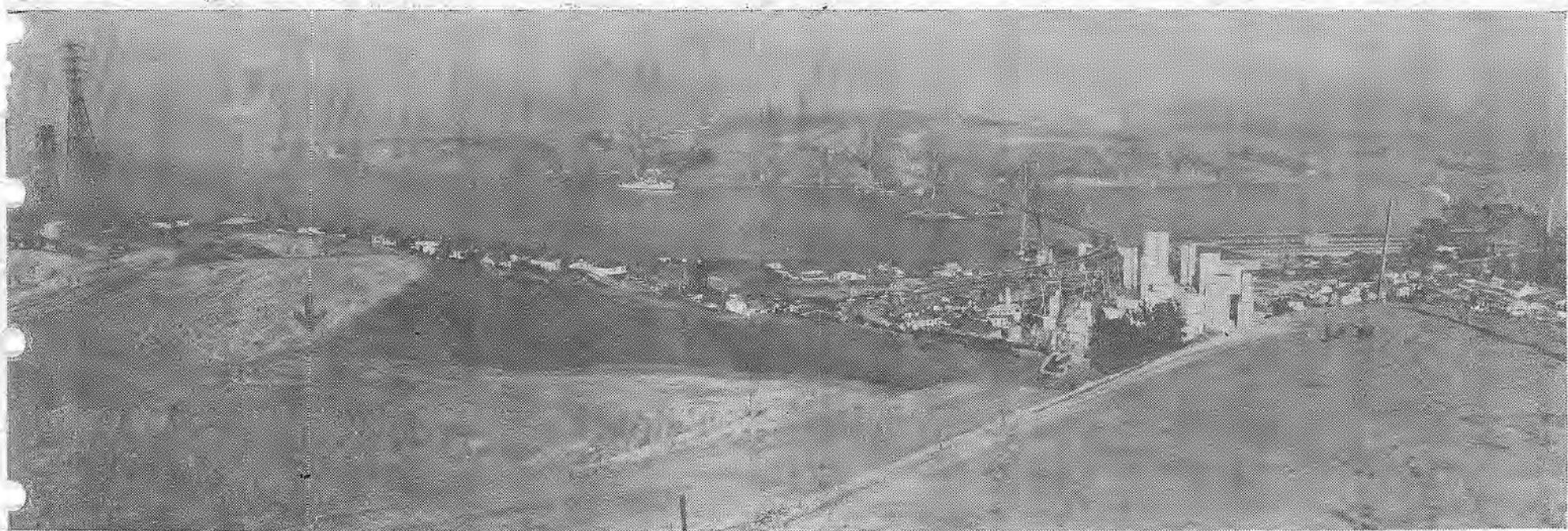
CARQUINEZ VS. CULEBRA.—Here you see the first slices being taken on the biggest whack at Mother Earth since the Culebra Cut in Panama Canal, the 300-foot canyon thru which Highway 40 starts a new career from the Straits to Bay Bridge. Engineers are sinking 300-foot shafts of concrete into the river-tidal currents down there to erect a twin to the present bridge, whose dogleg will be straightened a bit and run parallel to the new structure, whose giant, white pillars can be seen at lower right, near the town of Crockett and the G-H sugar plant. Arrow at right shows where they smack into the
