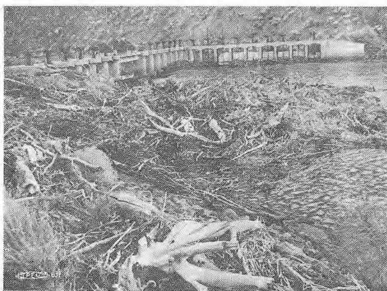
Millions of tons of water cascaded down steep eastern slopes of the Sierras in the Christmas flood and carried everything loose out onto the arid flats east of Reno. This log jam took out part of Derby Dam near Reno, but the break was quickly repaired by Engineers. (Pic by Joe Miller.)
