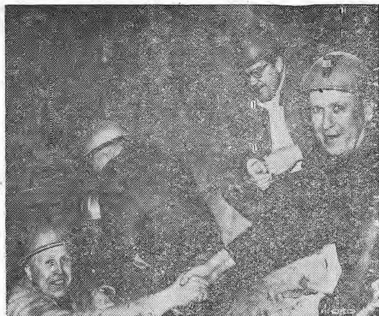
'HOLING THROUGH' RECORD —Deep inside Mount DuBose in British Columbia, Ted Leonard climbs over broken rock to shake hands with Whitey Davis as final blast joins two halves of 10-mile long Alcan Tunnel. The 18 AFL unions working on the project completed the "holing through" in 21 months to set a world's record for speed. (LPA)
