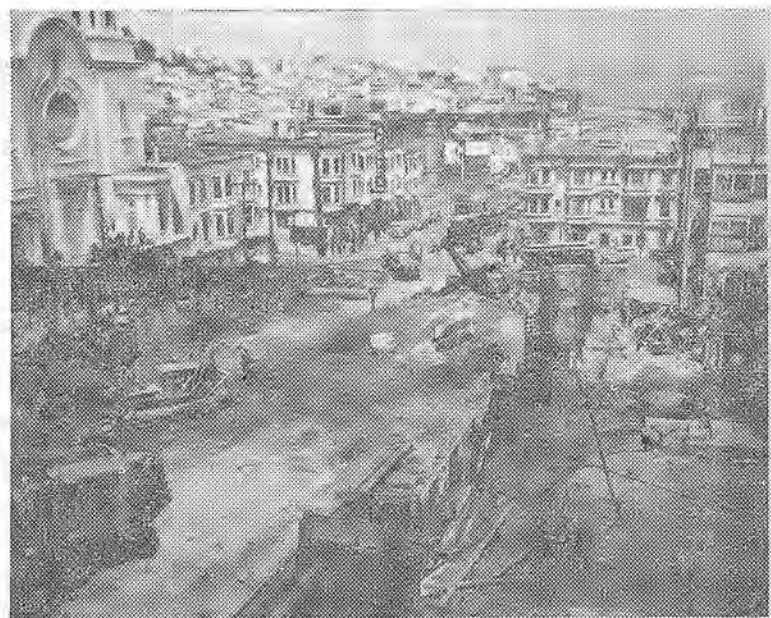
BEFORE AND AFTER . . . Shown above are two views of the site of the west portal of the new Broadway Tunnel under Russian Hill in San Francisco. At the left it is shown as it looked at the beginning of the project; at the right, as
