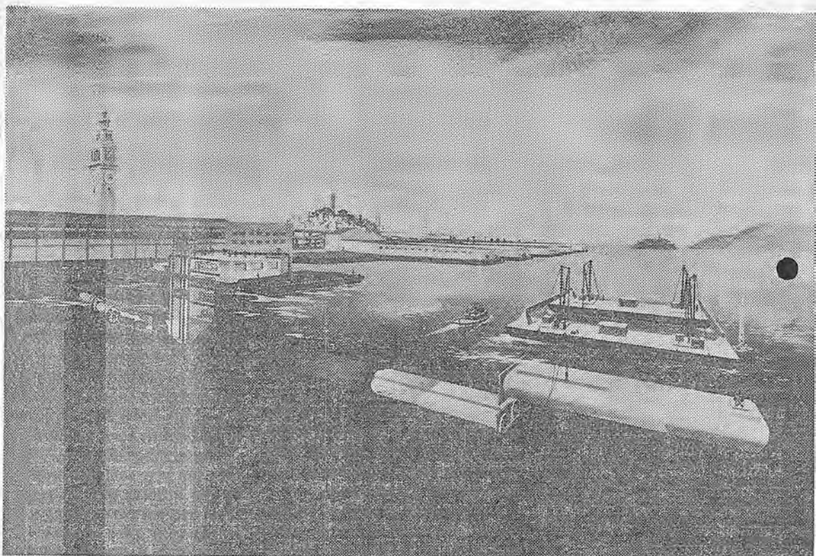
TUBE —Rapid Transit's artist conception shows how S. F. Bay submerged tube will be used in place to transport high speed commuter trains 6 miles beneath waters of Golden City. See story on construction below.
