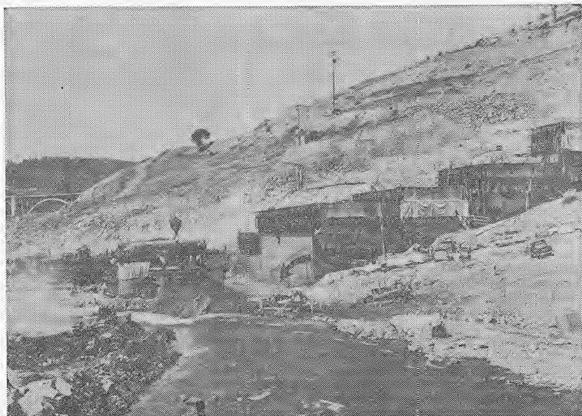
CLOSING THE GAP: First diversion of the Feather River for construction of Oroville Dam has been accomplished, and the river now runs through a gap between two of the core blocks near the right bank (shown by arrow). This photo was taken as dozers pushed fill from both banks to complete a dike which shunts the water into the desired channel. Work can now proceed on the center and left portions of the dam core block.
