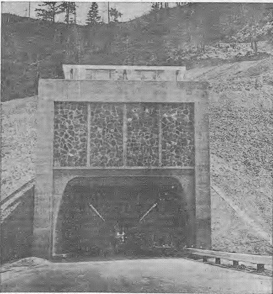
SHORTER AND QUICKER: This is the north portal of the new Randolph Collier Tunnel on Highway 199 through Oregon Mtn. on the California-Oregon border which was dedicated recently with appropriate ceremonies. It eliminates 2.8 miles of the old road with 128 tight curves and permits boosting the speed limit for this stretch from 25 to 60 miles an hour.
