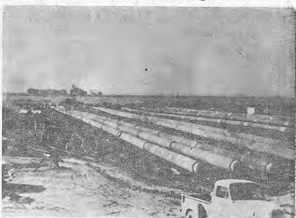
Pre-fabbed pipe ready to be welded together before being pulled across Sacramento River crossing at Antioch.
