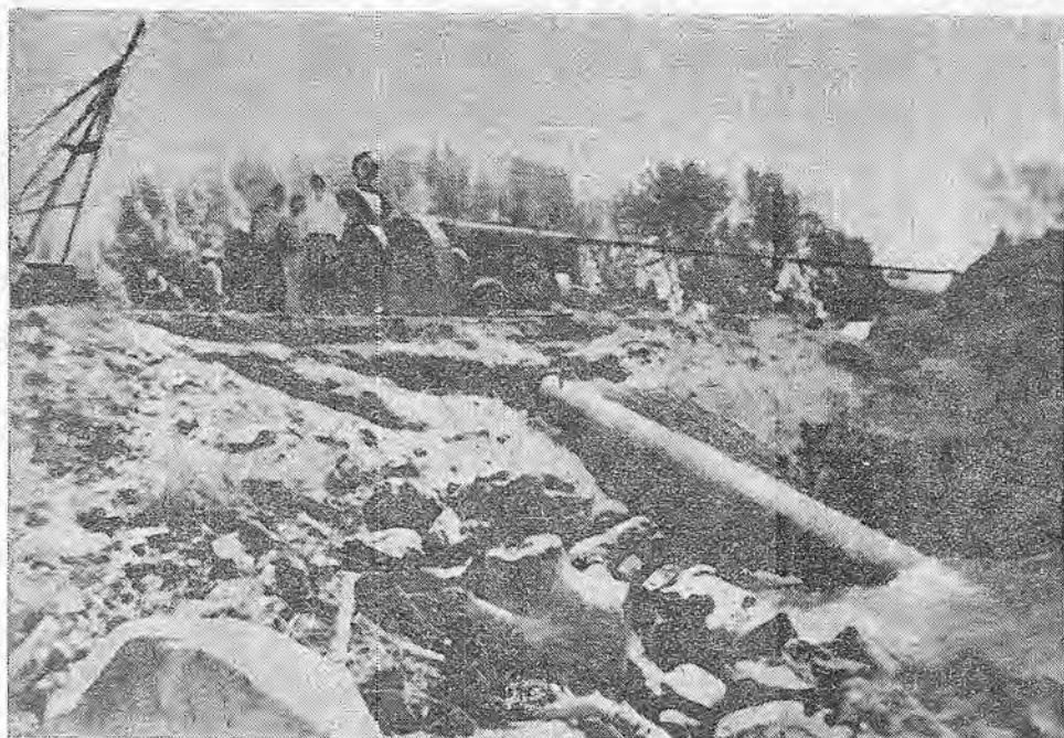
Two drum hoist which was used to pull pipe line across Sacramento River. First of such two lines is in place, with cable shown pulling the second line across.
