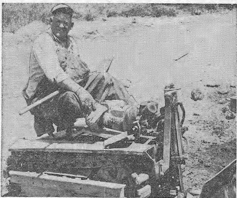
BIG SKINNER, SMALL CAT: No, this is not a picture of the latest thing for the scooter set. It's a picture of a man at work, Brother Herb Nefstead on an Agricat, grading for sidewalks on San Francisco's Alemany Freeway job.
