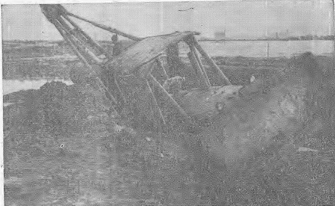
TRICKY GROUND: This D-7 boom Cat really got stuck in the mud on Hydraulic Dredging Co.'s job on the Sacramento deepwater channel. The operator was moving pipe sections in the spoil area, where the sandy surface may look okay but conceal mud pockets. This rig hit such a pocket and went in so deep it took three other Cats to drag it out.
