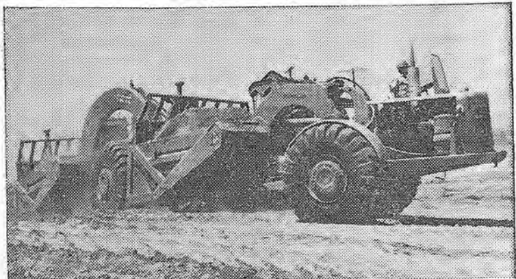
HARD AT IT . . . this multiple scraper is shown churning up Mother Earth on the California Aqueduct near Patterson.
