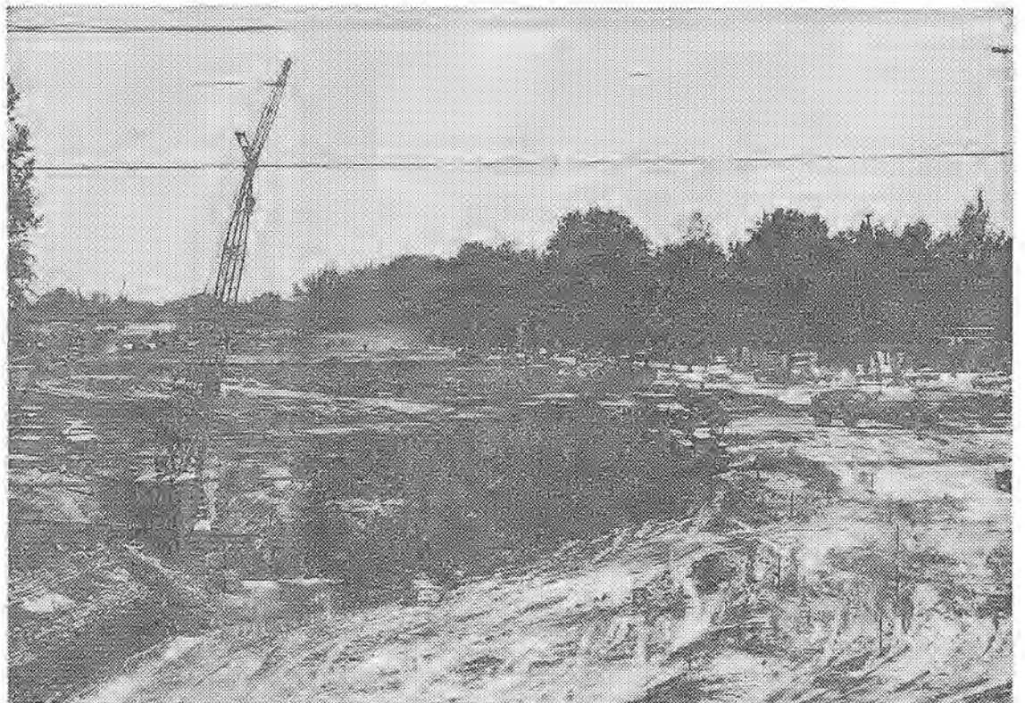
CAPITAL CITY . . . Sacramento is getting a new freeway and here looking south from the railroad overpass men and equipment are hard at it. Crane at left center is excavating for pumping station to handle runoff. Fill is being brought in by rigs in center.
