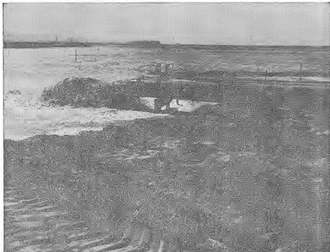
LIQUID LAND —This sand-filled water gushing from the end of a long pipeline shows how fill material is being pumped through pipes to fill in low-lying areas at Foster City. The water is subsequently drained off and fill remains. The method provides for fast, large-scale filling, results in excellent compaction for building sites, and eliminates the need for heavy trucking of earth-fill.
