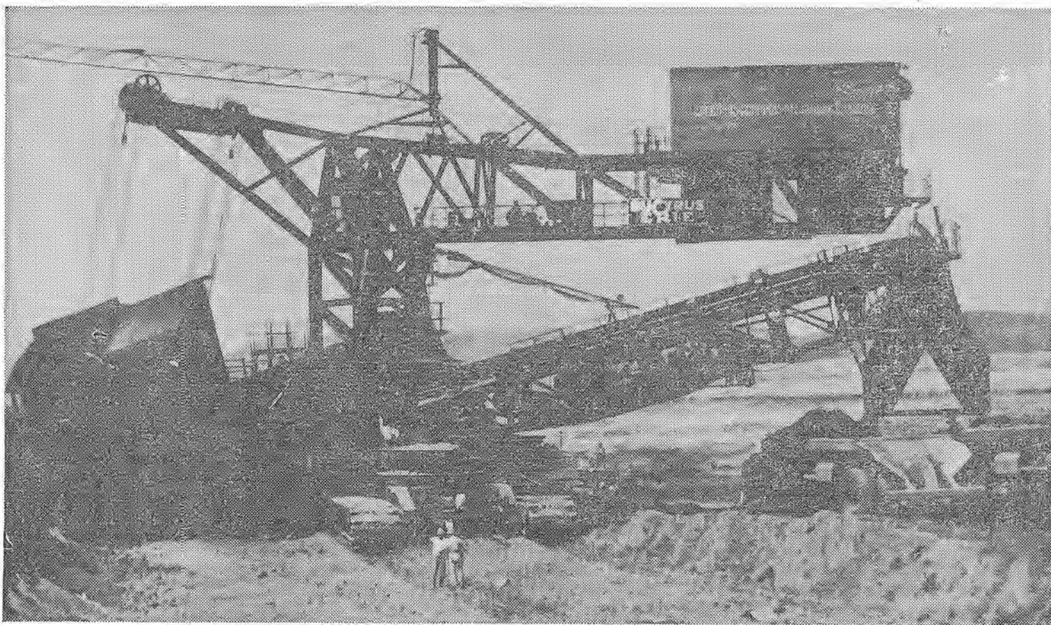
A WHOPPER . . . Here is the Los Banos "wheel" hard at work in over 100 degree heat. The Bucyrus-Erie Wheel is shown loading large belly dumps on one end while chews the material
