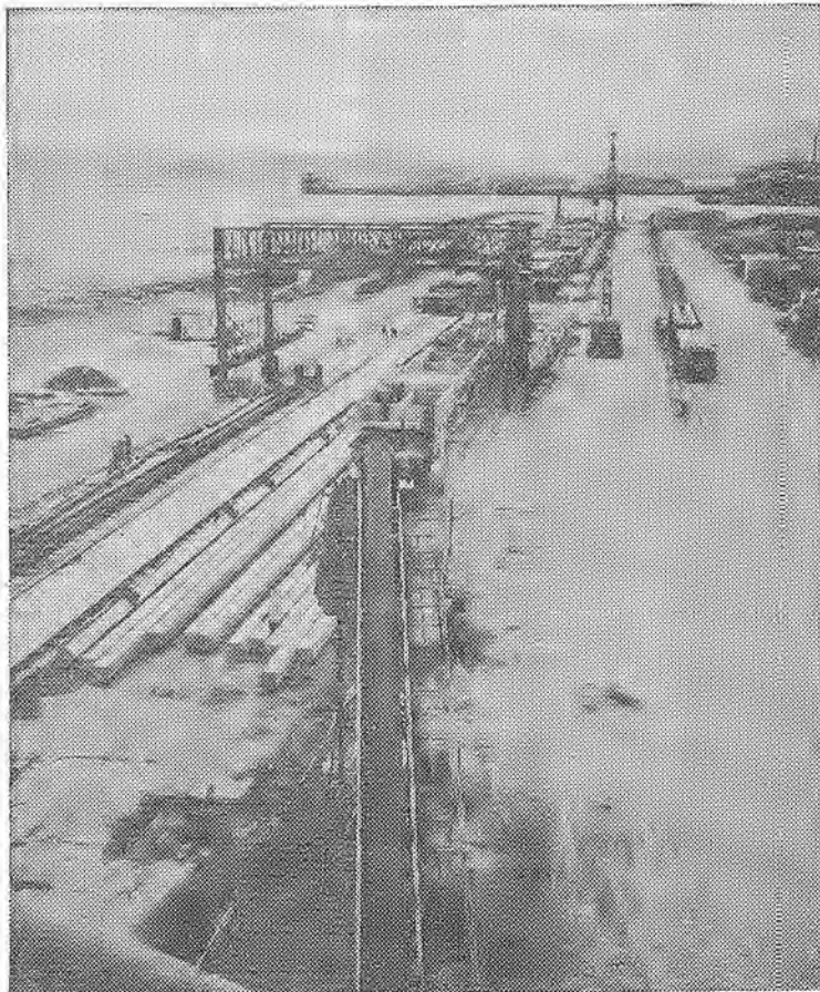
SPECIAL RIG —This special crane lifts 100 ton reinforced concrete pillars into place at the Bay Area Rapid Transit District test track near Concord.
