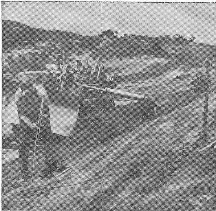
NEW SLOPER —attachment shown here to dozer is specially designed by Brother Jack McLean. Operator is Don Lawley with Jim DeBar using hand level on Green-Winston freeway near San Jose.
