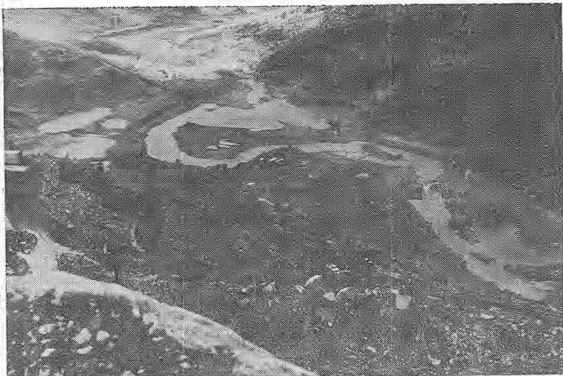
HELL HOLE —project on American River's Rubicon fork is seen here from helicopter loaned by Ets Hokin Construction Co. Earthfill dam gave away during December floods and is being re-filled. Same completion date is target of contractors.
