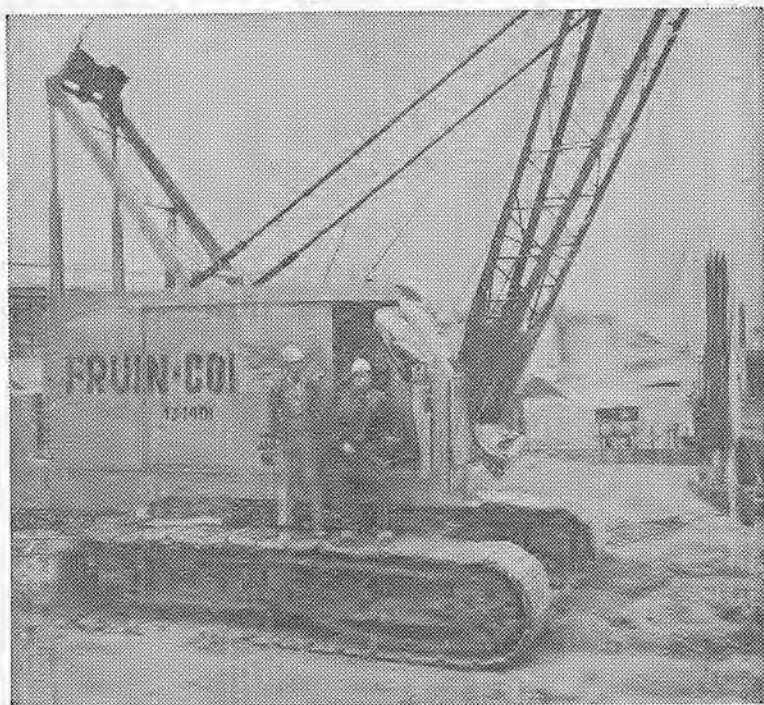
A NEW 60-TON American crane is pouring concrete on Fruin-Colnon's $3 million filter plant job for East Bay Municipal Utilities District. Proud of their "big baby" are Brothers John Cates (left), oiler, and Al Waltenbaugh, operator.
