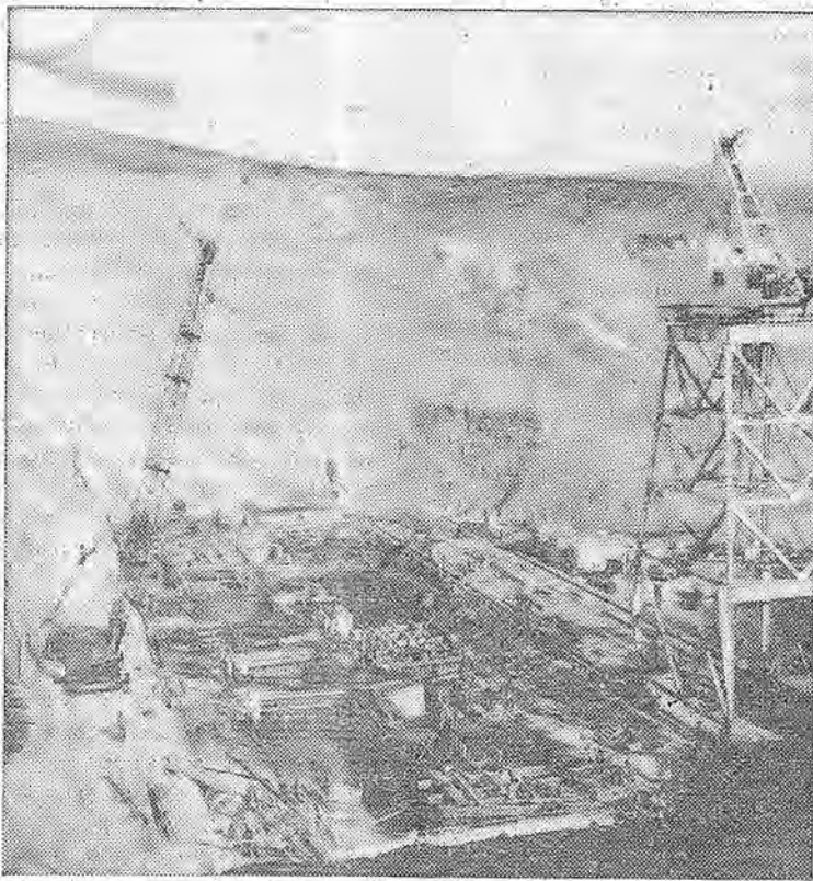
PUMPHOUSE . . . at Byron, Calif. shows a R-25 Whirly crane at right and an HC-108 ling belt, with 90 feet of boom and gib at left setting rebar and panels for Guy F. Atkinson Co.
