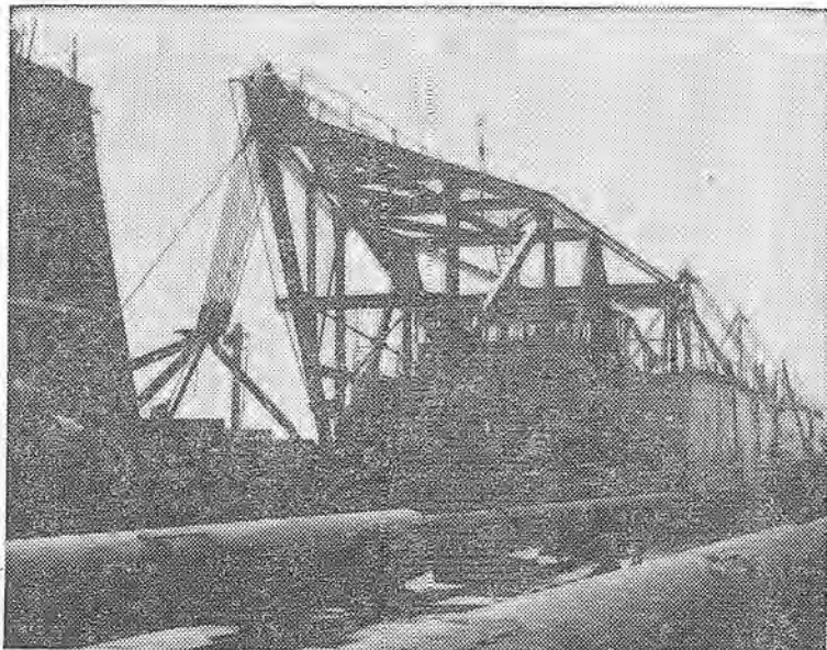
FROM THE FRONT —Here's a bow view of the double suction dredge built in Oakland by Associated Dredging Co.
