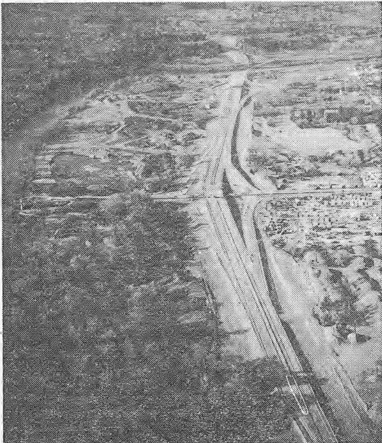
BIG JOB —Progress of the Harms Bros., B. C. Richter, H. Earl Parker, Lord and Bishop's highway 40 Alternate relocation job near Oroville is shown here. At center, underpass for the Oroville Lateral is nearing completion. Farther up the Montgomery Street underpass is taking shape. At the top is the Feather River crossing, where a new bridge is scheduled to be constructed. (Photo by Business Air Photos and Story Studio.).
