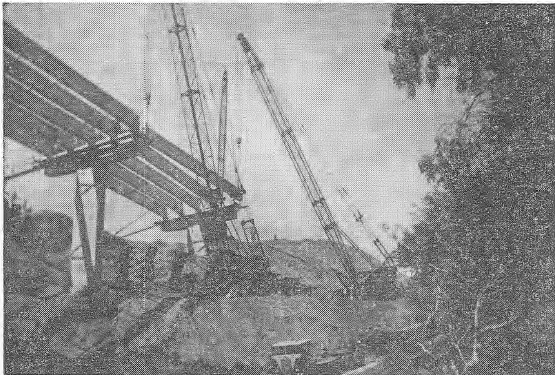
TUNITAS CREEK—THE DAN CAPUTO JOB 75-Foot, 24-Ton Concrete Beams; Kelly Bros. Rigs
