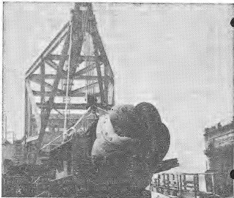
CUTTER —The rotating cutter-head for the mud unit is shown in this photo taken at the old Moore Dry Dock plant.
