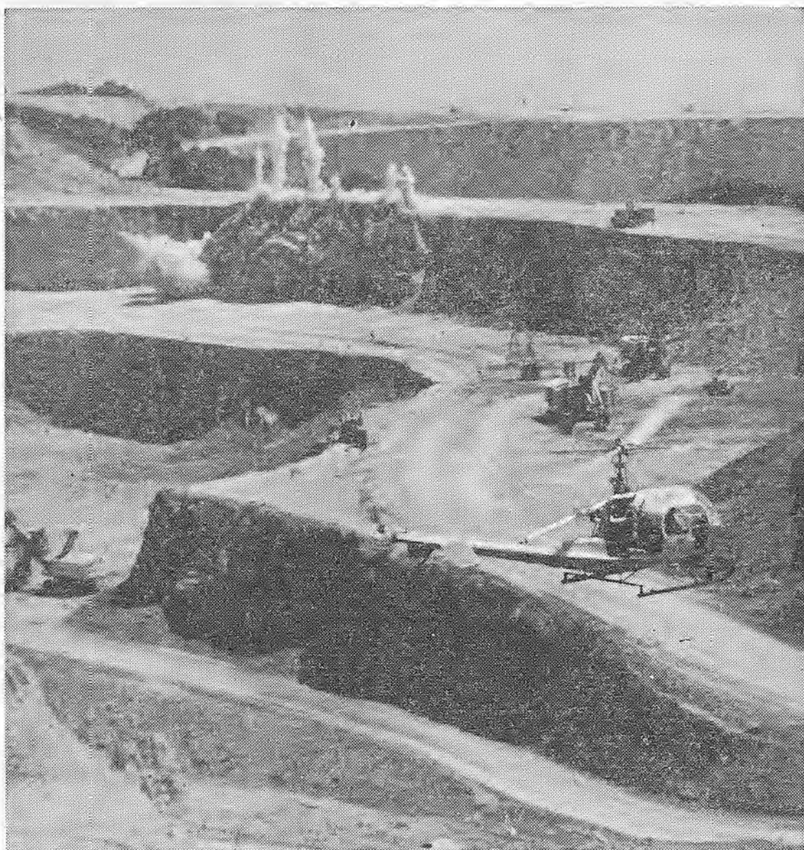
FROM THE AIR —Huge power shovels, each capable of a 5½-cubic yard bite, work in the terraced quarries of the Kaiser Permanente plant in the hills of Monta Vista, scooping up blasted limestone to provide the basic ingredient for cement.
