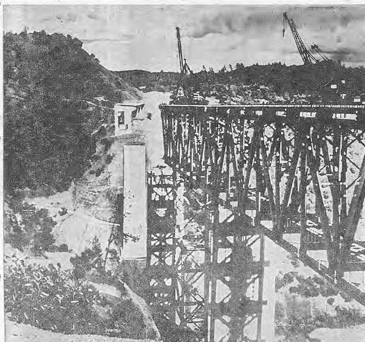
Stolte-Morrison-Knudson Company is approximately 60 per cent completed on the construction of the West Branch River Bridge near Oroville. This is part of the relocation work on the Water Resources Development System. The double-deck bridge
