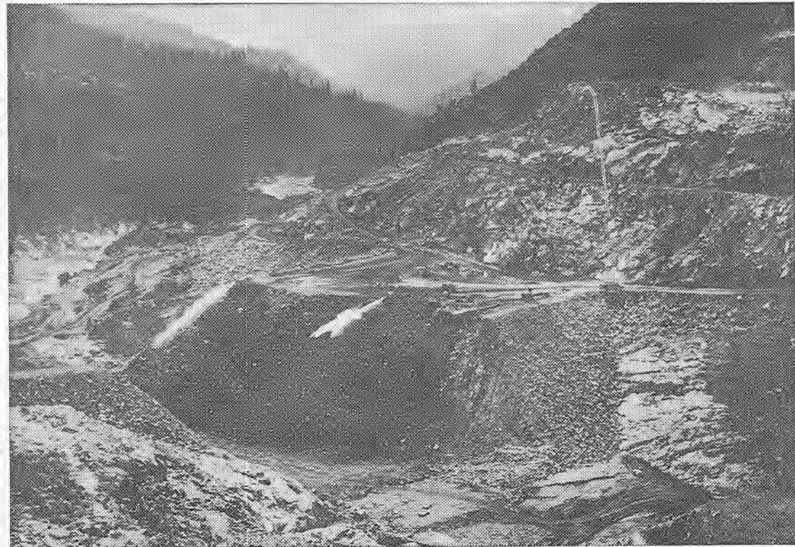
REBUILDING DAMAGE . . . winter floods washed out Hell Hole Dam on the American River project causing over $100 million in damage. The big pic-
