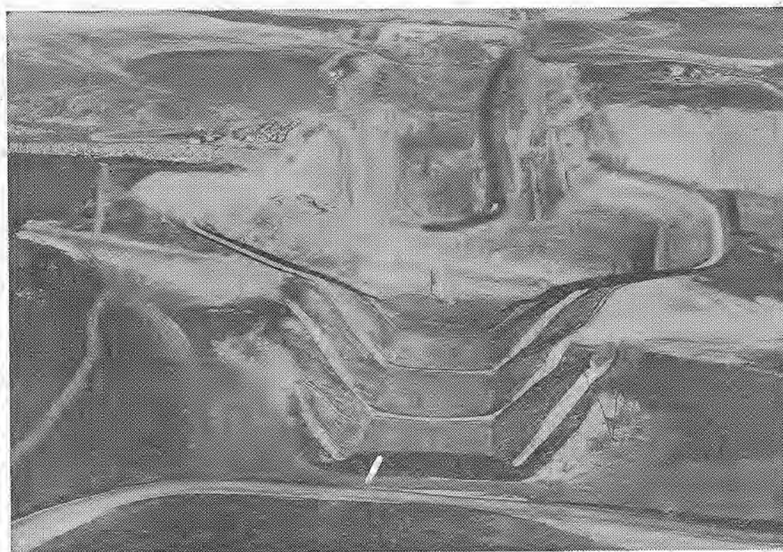
AERIAL VIEW . . . the intake channel on the California Aqueduct Canal project near Byron. This is part of the State Public Water Resource Program to develop the California Water Program. Work is being done by Peter Kiewit, moving over 11 million yards.
