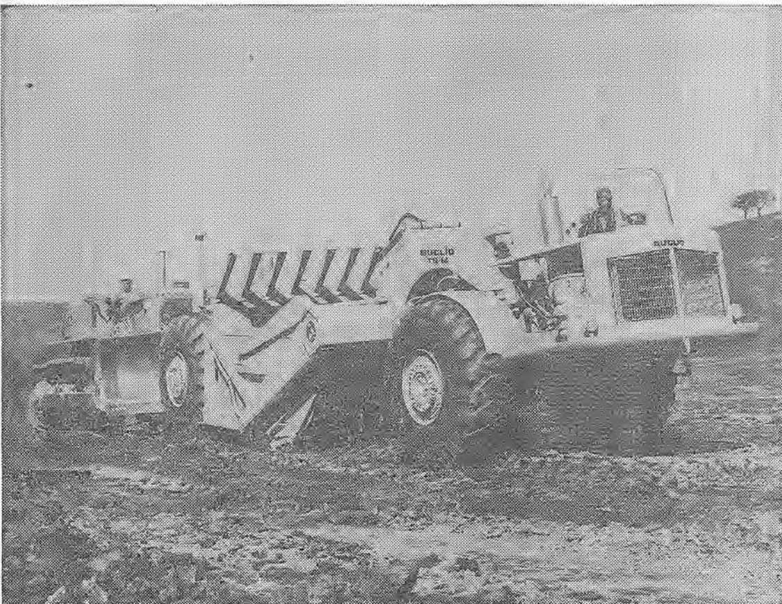
LEARNING HOW . . . This Euclid TS-14 scraper, with an assist from a D A Cat is being propelled up a hill at Camp Roberts by an Engineer trainee.
