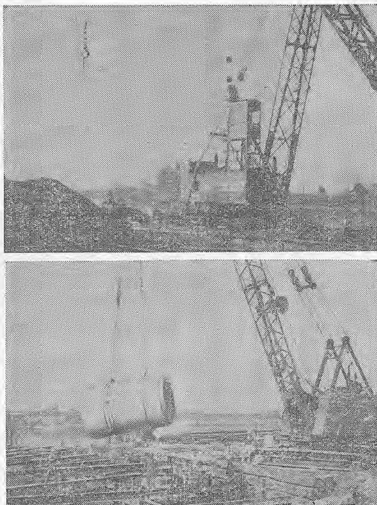
CROSSING THE RIVER: Carrying a pipeline across the San Joaquin River on the Healy-Tibbetts-Graver job in the Stockton area. Top photo shows derrick barge with Bros. Bob Miller operating and Lloyd Edwards oiling, clamping for the pipe bed on the east side of the river. Bottom photo: a 3900 Manitowoc on the other side, with John Dorton operating and Lewis Moody oiling, placing the pipe.
